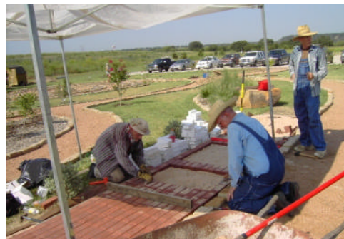
Volunteers installing the first brick sections
